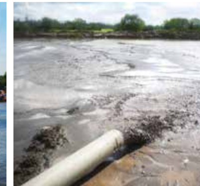
LEFT PAGE: Deep aluminium fins as passive sun-shading feature; BELOW FROM LEFT: Transporting sand with barges to site; pumping a mixture of water and sand from barge to site which was originally part of the body of a river
