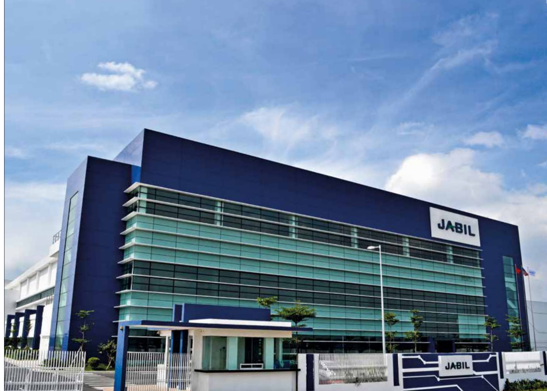
View of the building from 'Duong D1'
