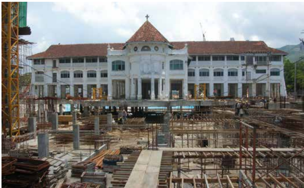
The construction involved the introduction of new micropiles and ground beams to underpin a new transfer slab that supports the entire structure
